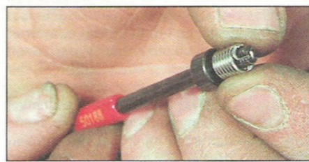
2.28 ... fit insert on the installing tool ...
